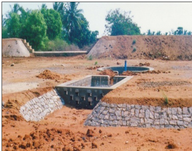
Figure 2: Recharge shaft in percolation pond
