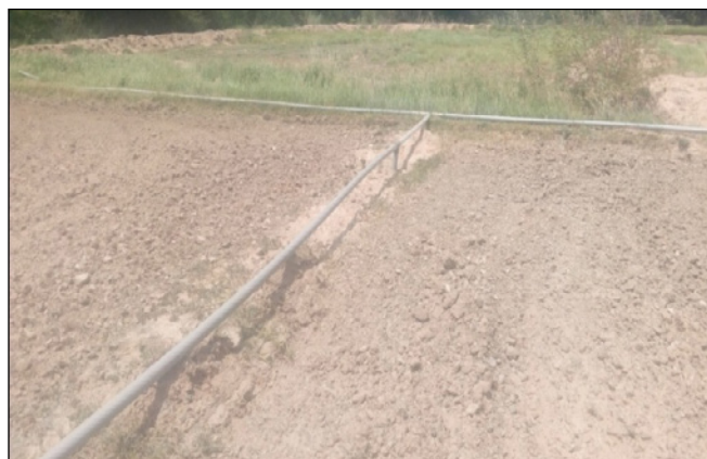
Figure 4: Installation of sub irrigation system
