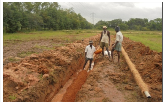
Figure 3: Installation of controlled drainage
