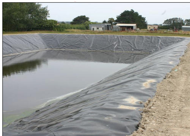
Figure 1: Farm Pond with lining (Courtesy: Ocean Non-Woven Pvt Ltd., Delhi)
